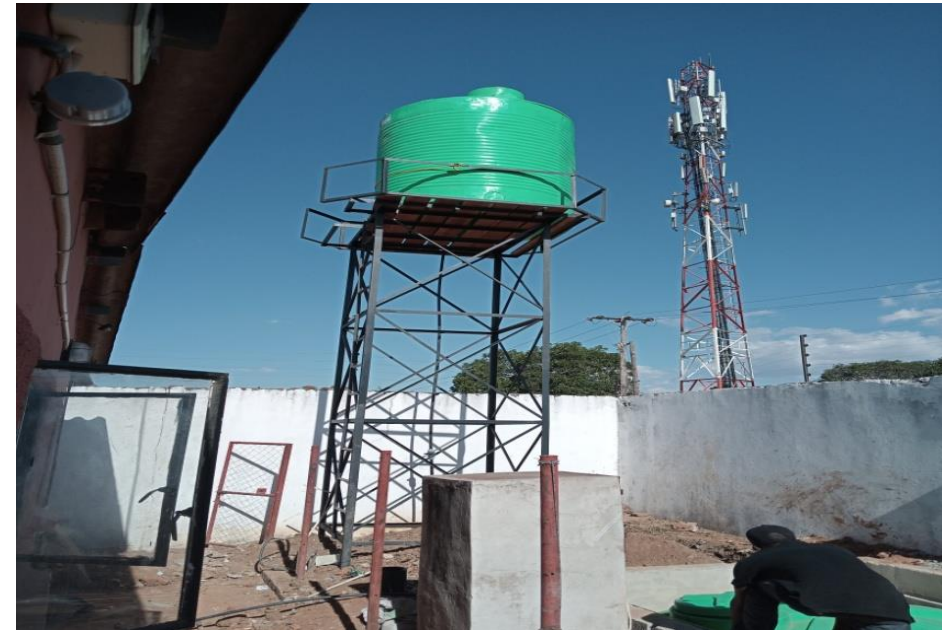
Above, Installation of water reticulation system at School.
