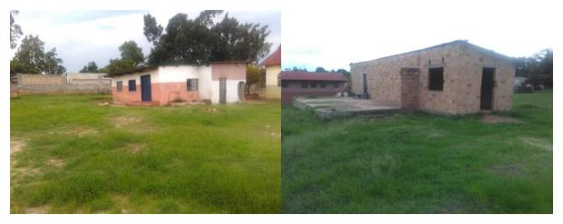
Front and rear of the kitchen. Kitchen requires doors and frames, window panes and frames and plastering as well as piping to be connected to the borehole.
