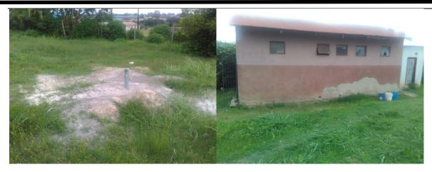
Borehole and ablution block requiring piping and plumbing works. Ablution also requires plastering and cleaning materials.
