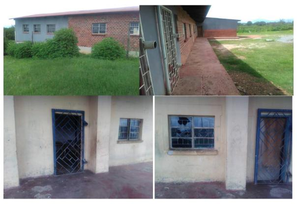
Classrooms requiring plastering, repair/replacement of grill doors and doors and replacement of broken windows.
